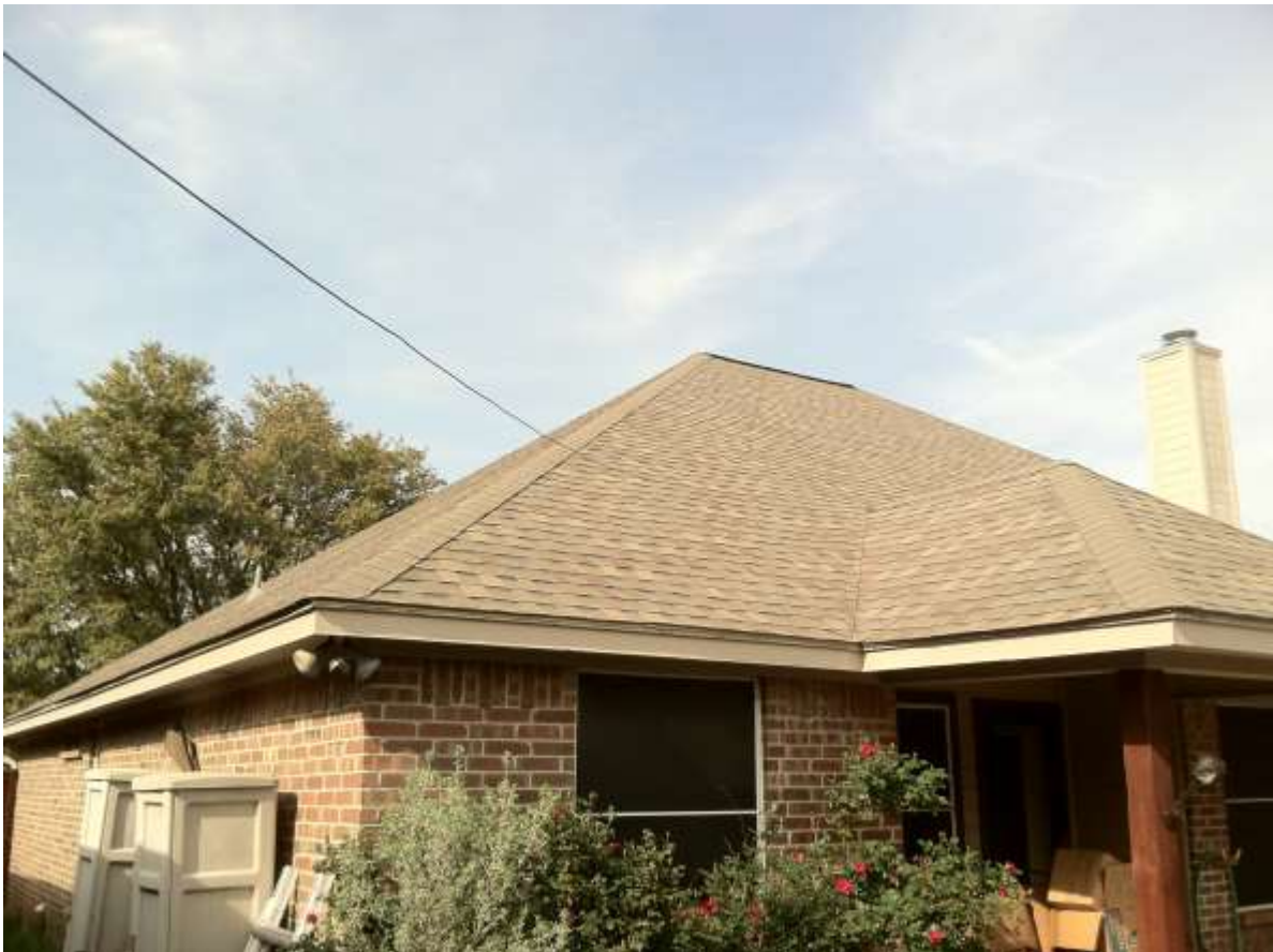
View from Southwest UNUN to Roof Apex Showing Low Visibility
