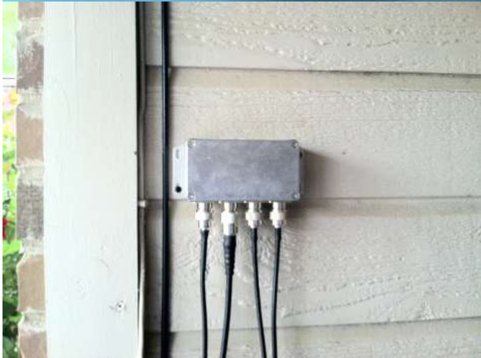
Antenna Switch Construction and Mounting
